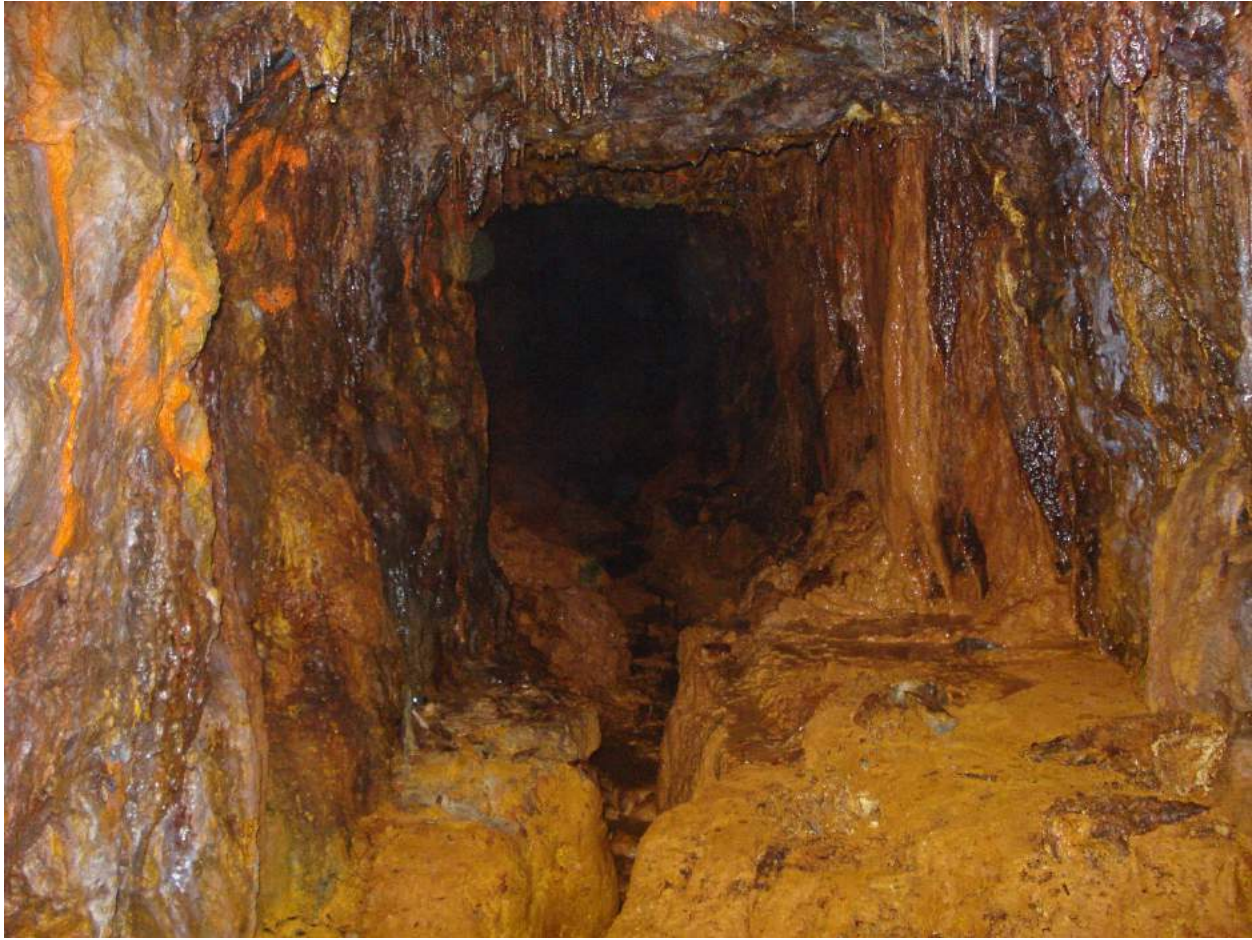
FIGURE 16 SHEAR B EXPOSED IN THE 5 LEVEL DRIFT SHOWING FE-OXIDATION DUE TO PERCOLATING GROUND WATER (O'BRIEN, 2011)
