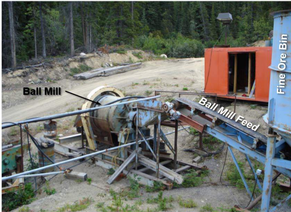
FIGURE 64 BALL MILL AND HOPPER
