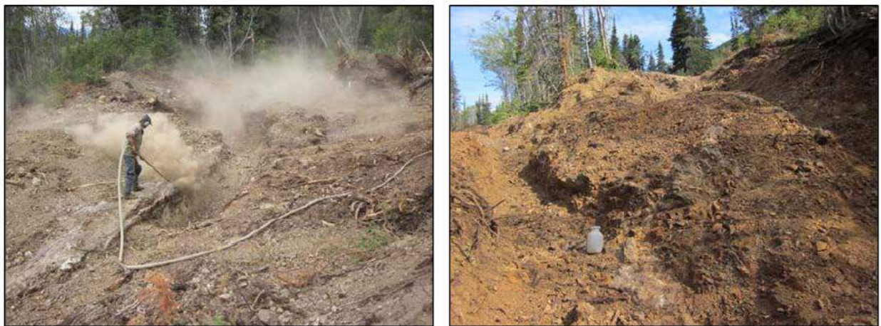
FIGURE 26 TRENCHES WERE EXCAVATED AND CLEANED OFF WITH A BLOW PIPE PRIOR TO MAPPING AND CHANNEL SAMPLING
